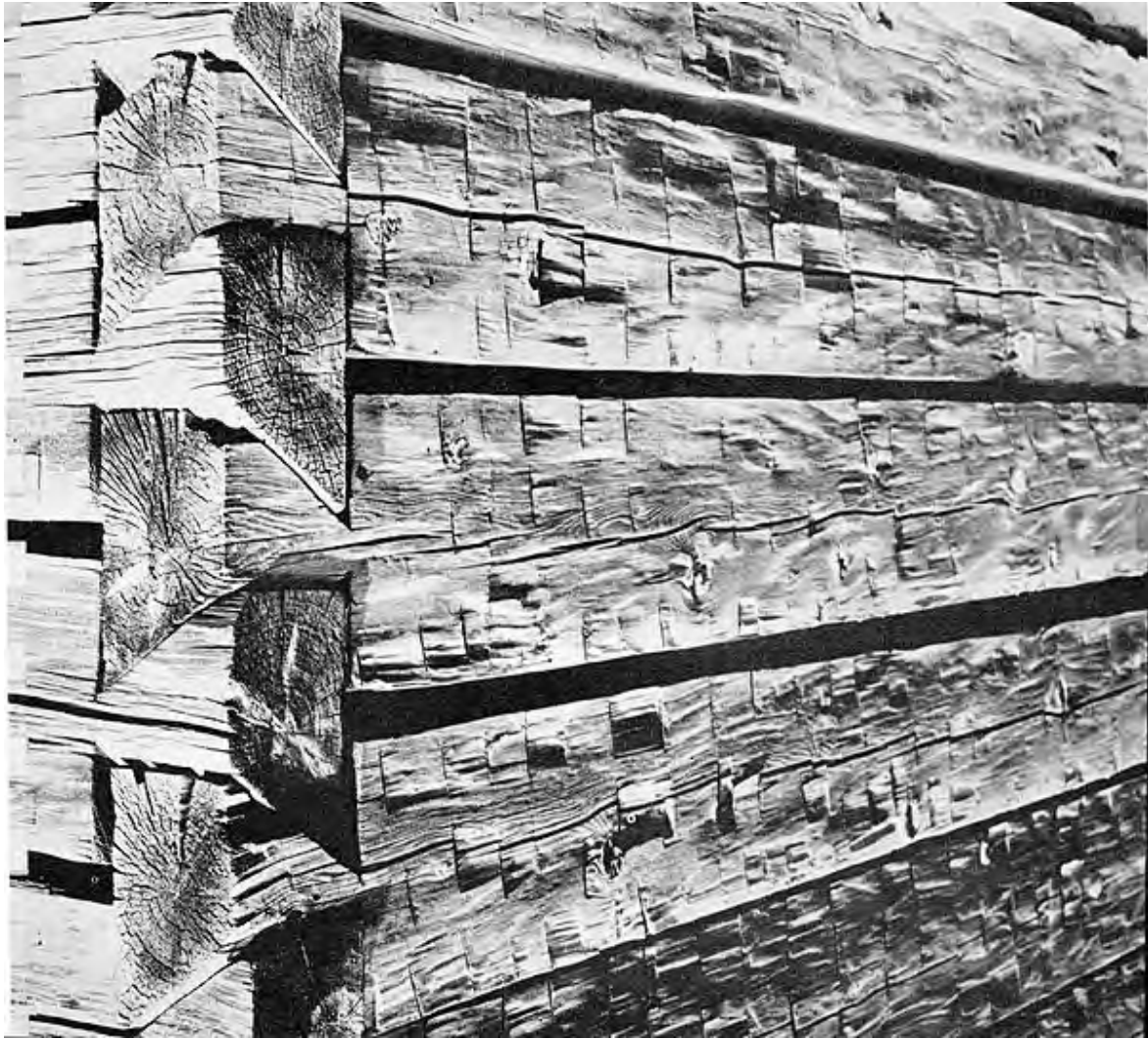
Mortised triangle corners on school, date unknown. Siskiyou County Office of Education School History Collection.
