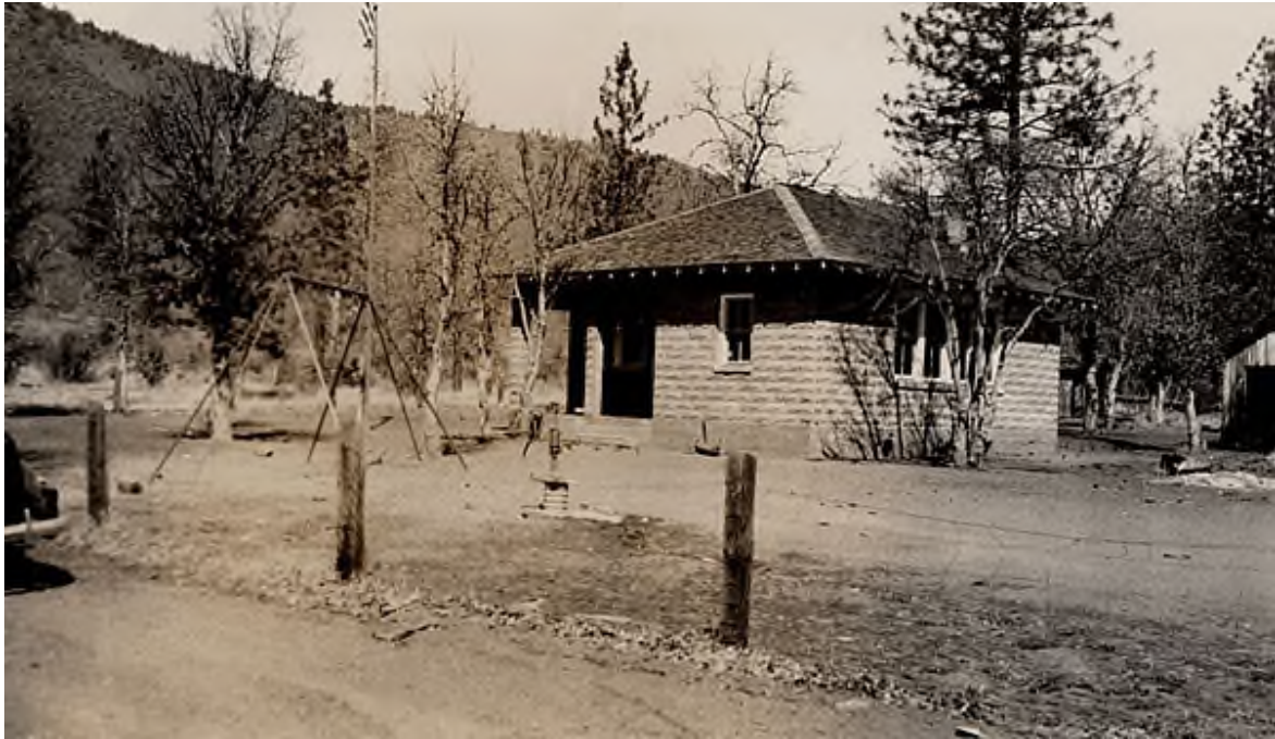
ca. 1939. Photo by Mildred Grant, donated by Roderick and Larry Grant. This school building was one which could be ordered from the Sears and Roebuck catalog and then assembled on site.
