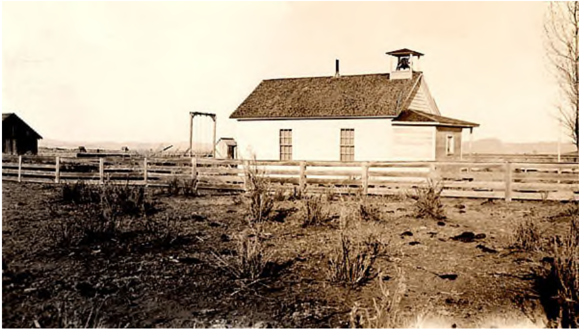
Oklahoma School (aka. Oklahoma Emergency School), ca. 1939. Photo by Mildred Grant, donated by Roderick and Larry Grant.
